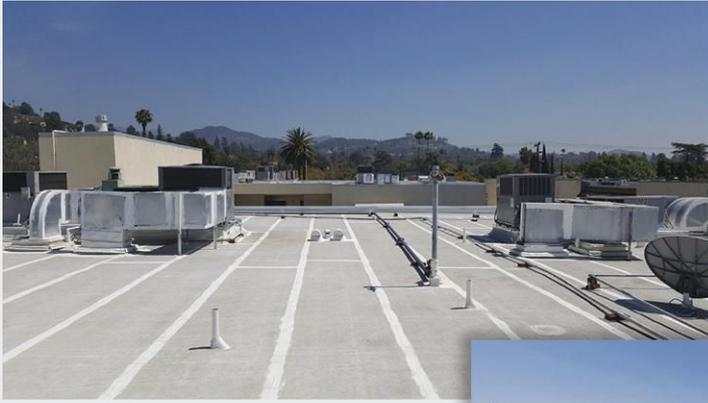
➤ ADCO Roofing and Waterproofing installed a new, highly-reflective roof system on the Campbell House HOA building in Glendale, Calif. For the cap sheet, the contractor used 17,000 sq. ft. of Polyglass' Polyfresko® G, a white modified bitumen membrane that has improved granule adhesion and is resistant to puncture, stain and UV.
